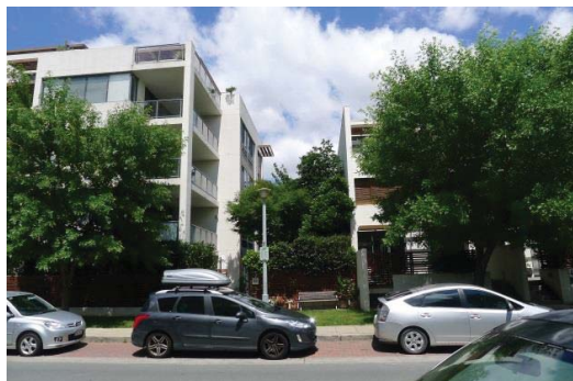
40. Pedestrian right of way Source: THSC
