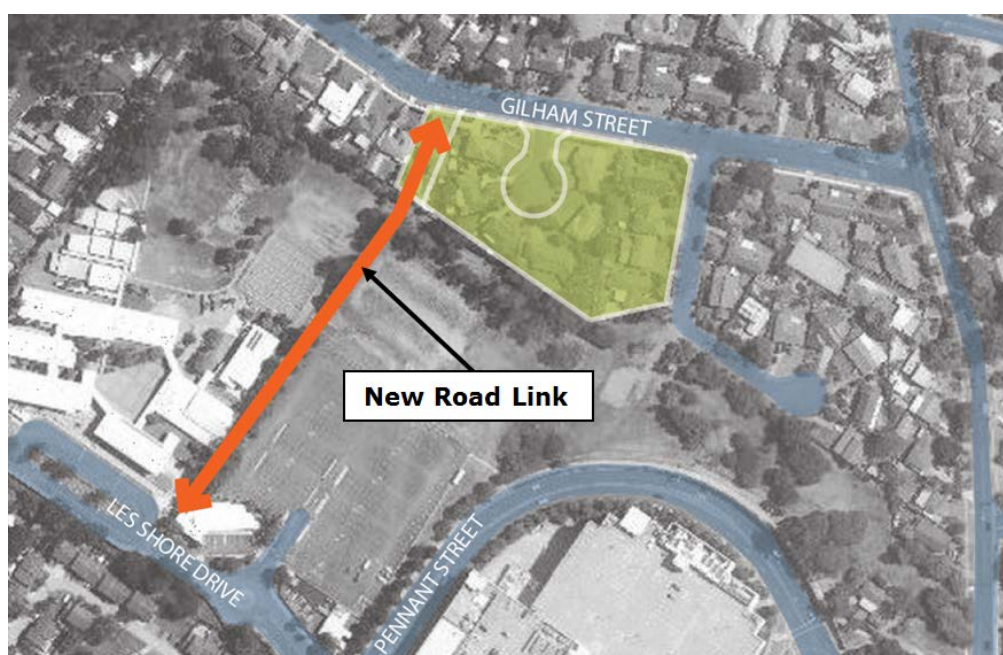
Figure 12 Future Road Link
