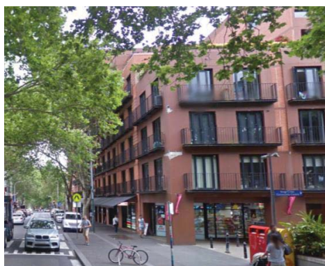
4. Retail at ground level Source: Google Streetview
