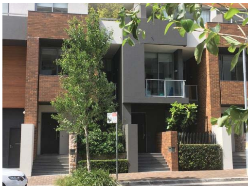
46. Terrace style housing with access to street. Source : THSC
